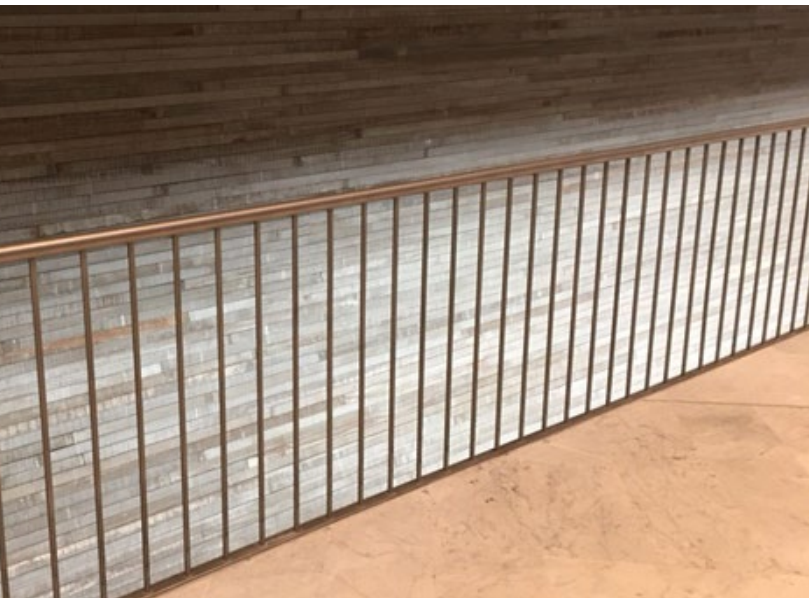
Bauhaus - Museum Dessau. Use of brass to refine the appearance of standard compliant balustrade.
