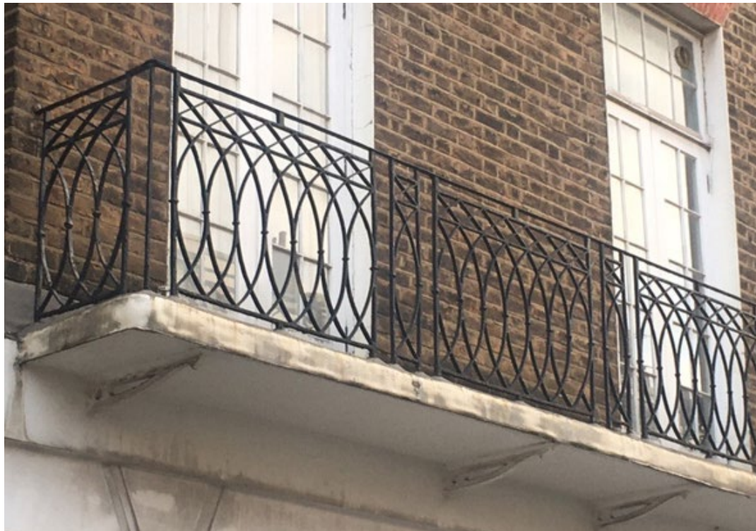
Georgian, London, restrained use of wrought iron.
