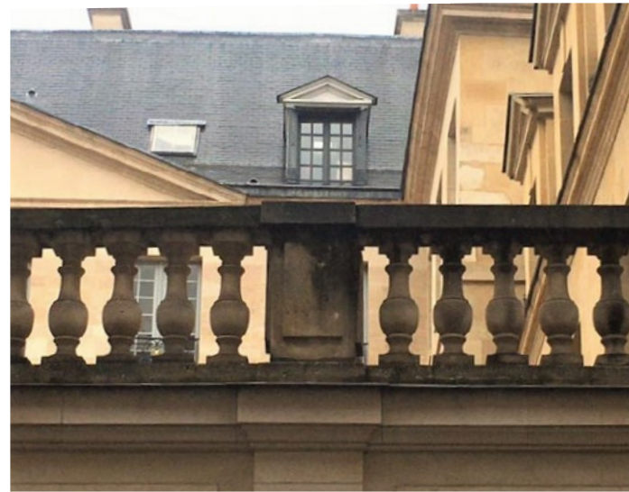
Typical limestone balustrade, Paris.
