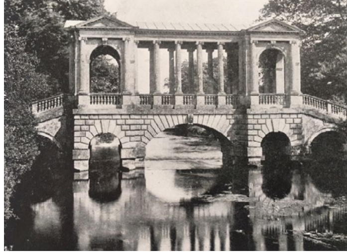
Safety on public structures encouraged balustrades, with reinforcing pillars.
