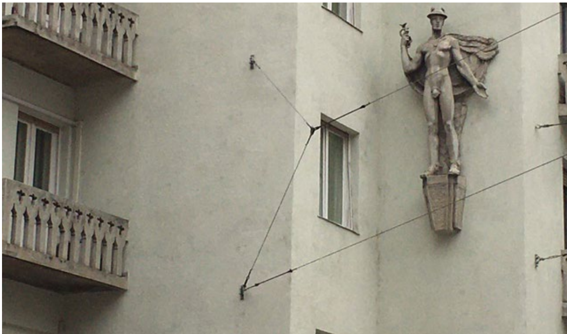
Perforated screen design balustrade - Budapest
