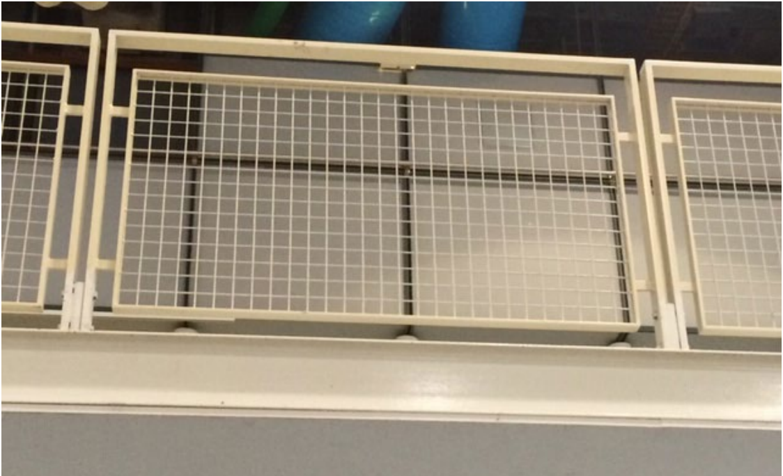
Centre Pompidou - Piano Rodgers. Handrail follows the prefabricated aesthetic.
