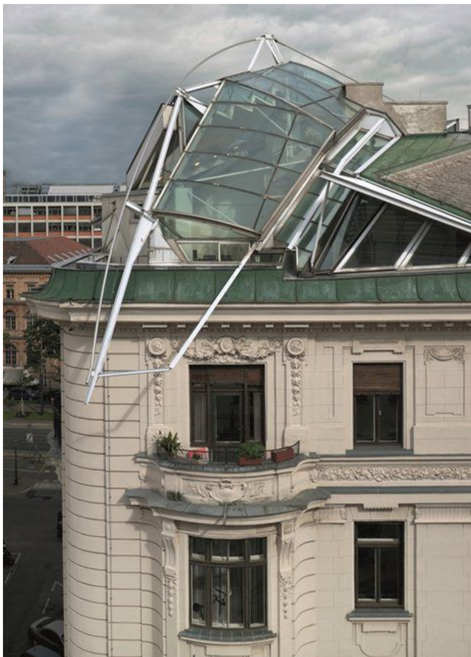
Falkestrasse Apartment in Vienna by Coop Himmelb(l)au
